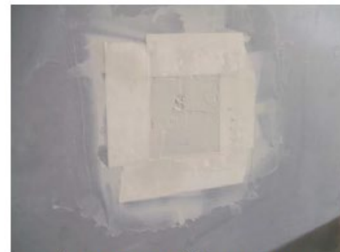
Figure 5: Tape and Finish Patched Area
