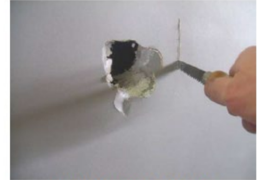
Figure 2: Square Off Damaged Area
