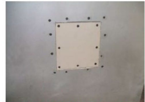
Figure 4: Apply Gypsum Panel Patch
