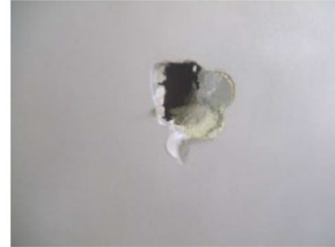
Figure 1: Damaged Gypsum Panel
